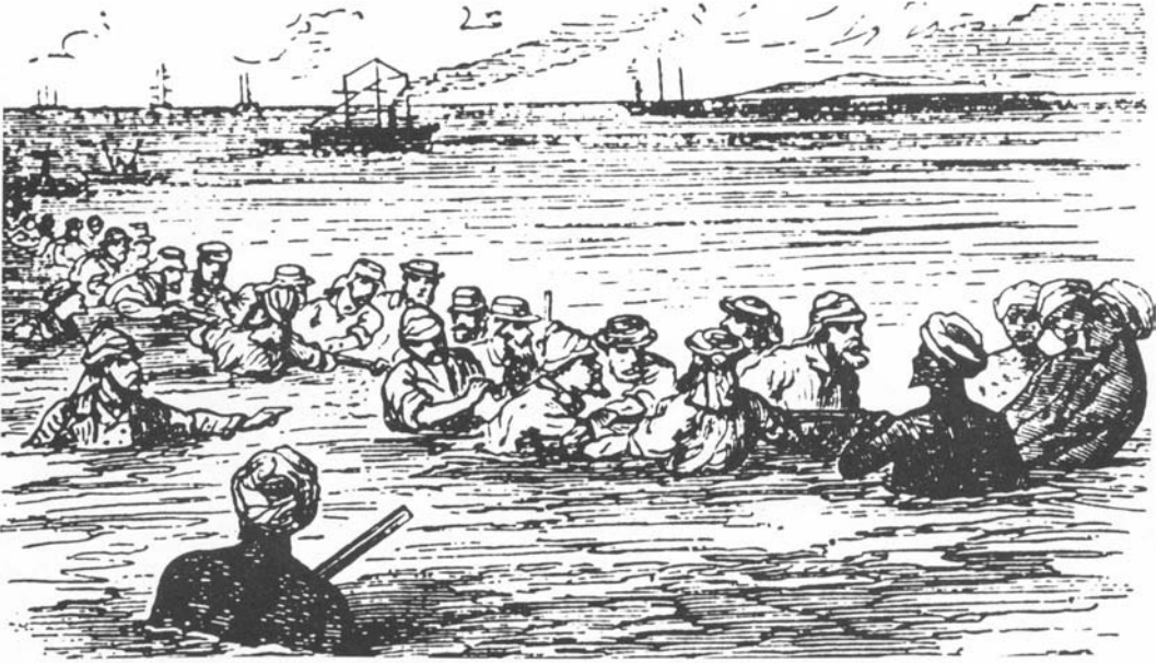
Figure 15.2 The shore end of the Persian Gulf cable being landed through the mud at the mouth of the Shatt al Arab in 1864. Sir Charles Bright, who directed the operation, is pictured at left with his arm outstretched. Completion of this cable, along with connecting landlines through Turkey, Mesopotamia, and Pakistan, provided a vital link from Britain to India. (From Bright 1898, 73; based on an engraving originally published in the Illustrated London News , 1864.)
